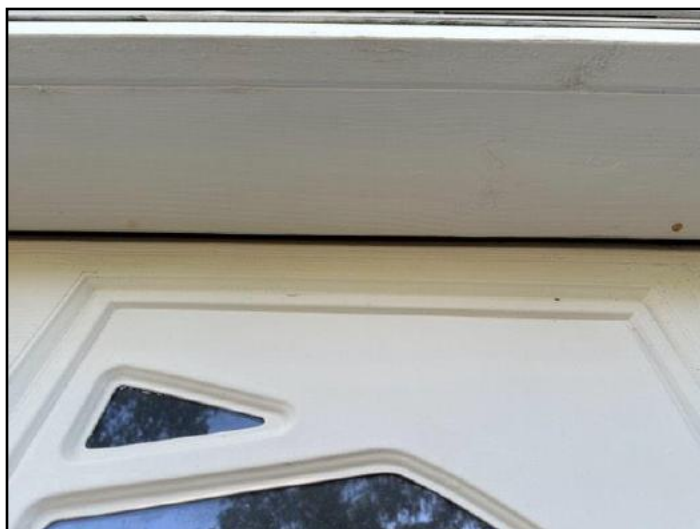
25. Weatherstripping damaged or missing.
