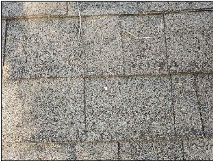
1. Granule loss is an indication of roof...
