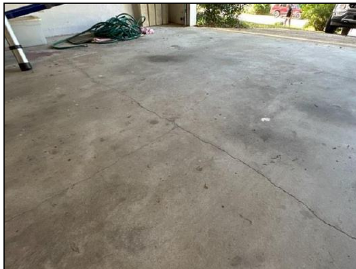
84. Garage floor has typical cracks but appears...
