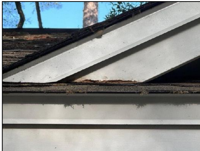
65. Observed wood rot or Detected above normal...
