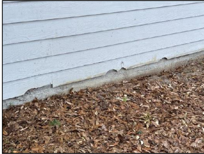
76. Cracked, split or broken
