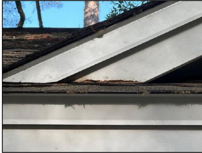
8. Observed wood rot or Detected above normal...
