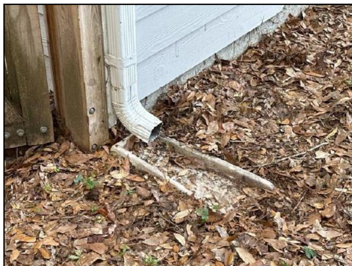
5. Gutter discharge 4-6 feet from building or...
