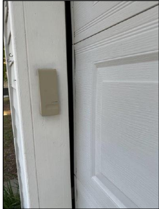
86. Weatherstripping damaged or missing.
