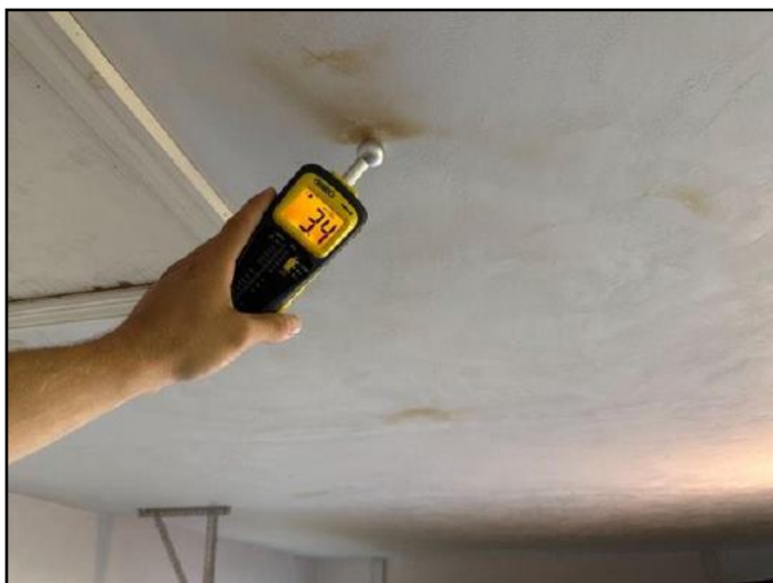
35. Stains on ceiling. NO moisture detected...
