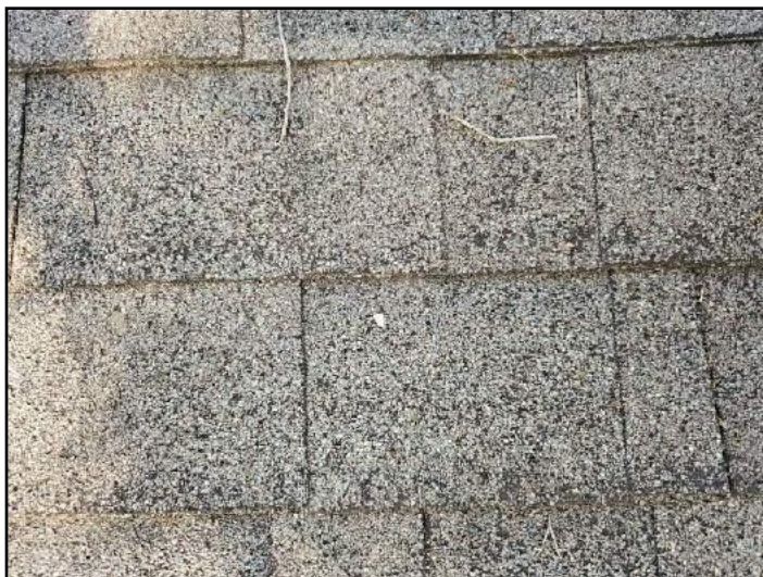
42. Granule loss is an indication of roof...
