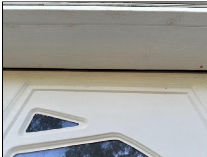
87. Weatherstripping damaged or missing.
