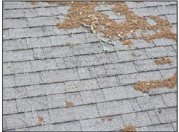
2. Granule loss is an indication of roof...
