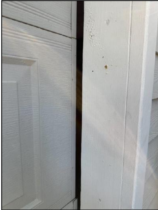
85. Weatherstripping damaged or missing.
