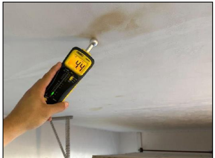
163. Stains on ceiling. NO moisture detected...
