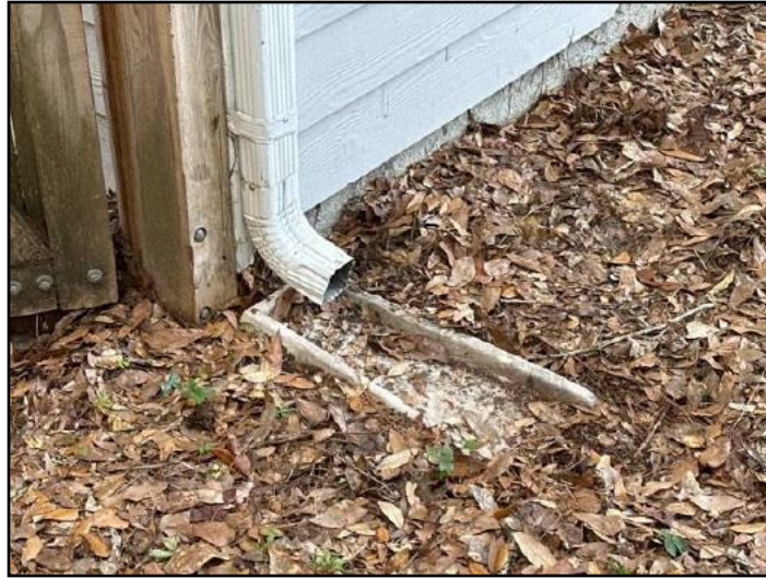
62. Gutter discharge 4-6 feet from building or...
