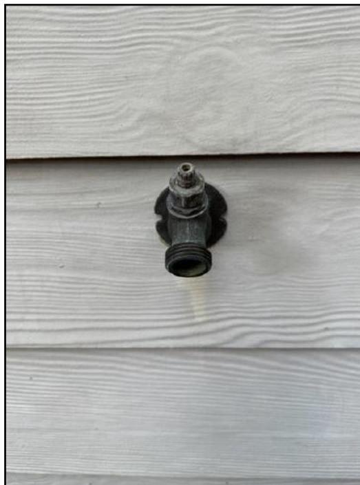
31. Mechanical damage
