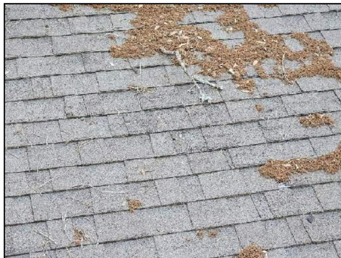
43. Granule loss is an indication of roof...
