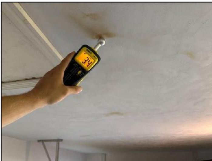
162. Stains on ceiling. NO moisture detected...
