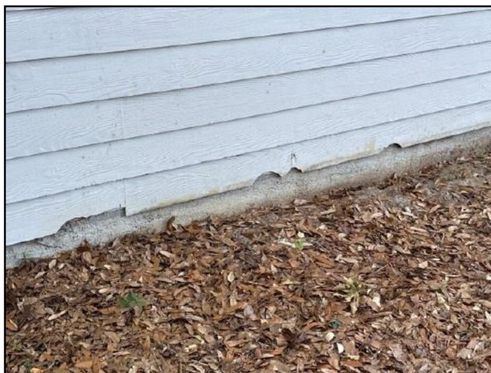
19. Cracked, split or broken
