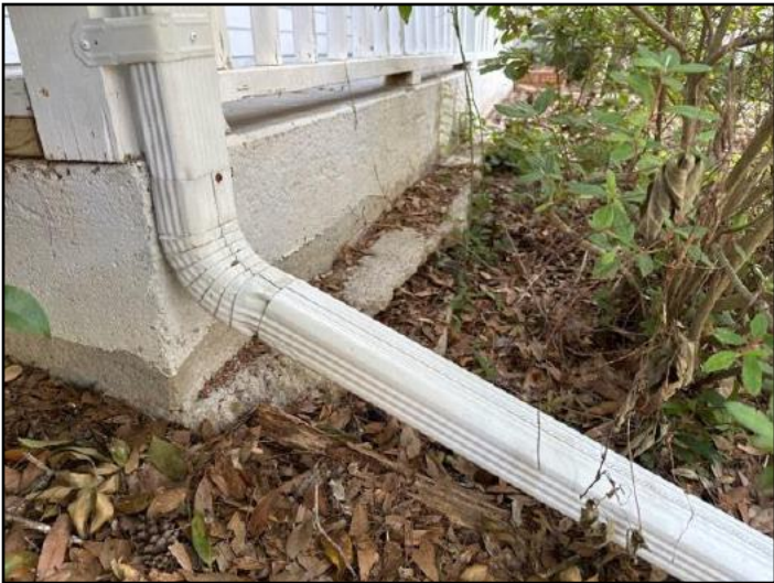
90. Soil erosion noted. This condition can...
